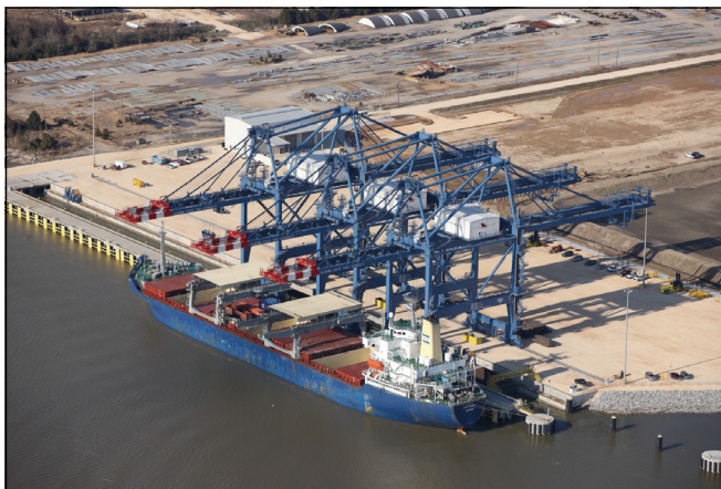
The steel slab terminal at Pinto Island, Mobile, Alabama, with barges between the crane legs loaded directly from the ship, is seen by Dr Ashar as a good illustration of the PTP concept. (The barge indexer can just be made out on the left)
